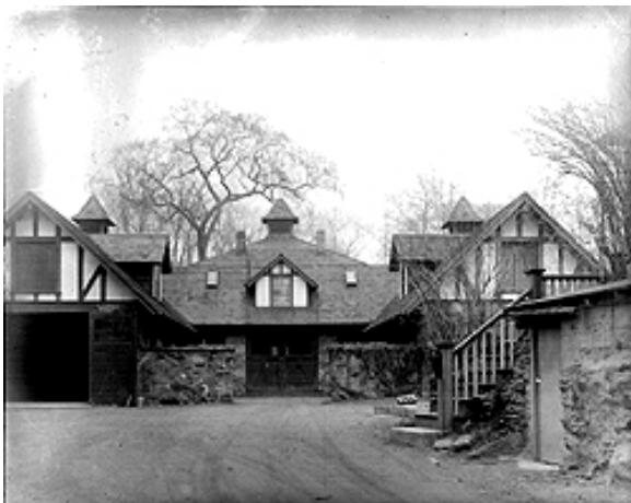
Stables of the Bolton Priory on April 2, 1938 Prior to Conversion Into Residence During the 1950s; Bolton Priory is Listed on the National Register of Historic Places
