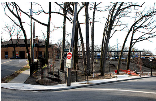
Town of Pelham Memorial to Town's Victims of September 11 Attack Under Construction with Pelham Train Station in Background.
