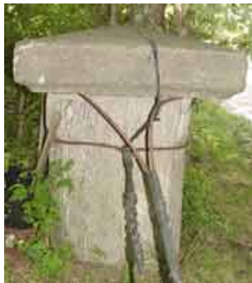
West Pillar, Shore Road
