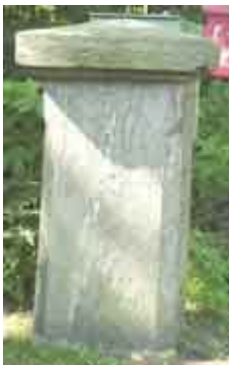
East Pillar, Shore Road
